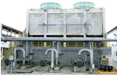
Figure 2 Cooling tower
